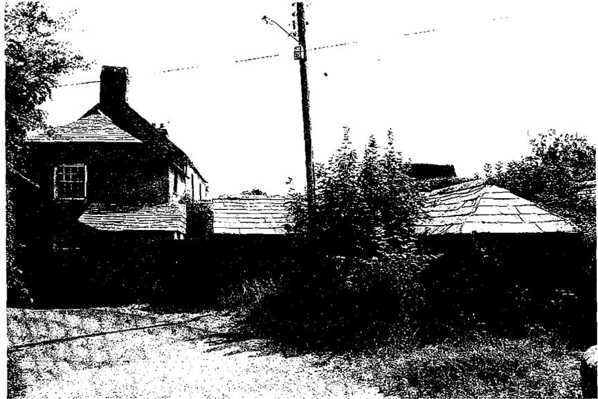
*Several pig houses survive in a relatively unaltered state. Rag slate roofs with mitred hips and red clay ridge tiles are a traditional detail.*
