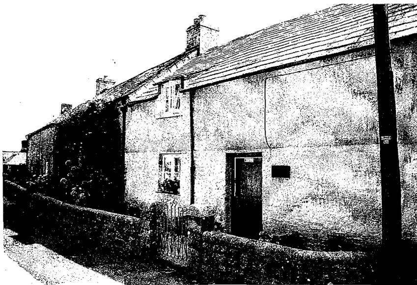
*A stone and cob cottage typical of those in School Lane. Simple side hung casement windows, wicket gates, wedge shaped dormers and stone boundary walls are traditional vernacular details, as is the slate wind spur course at the gable verge of the adjoining house.*
