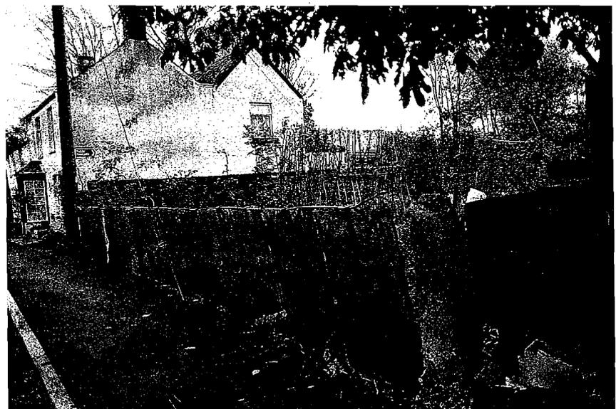
*Garden boundary walls in St Tudy are sometimes formed by massive Delabole slate slabs laid on end.*
