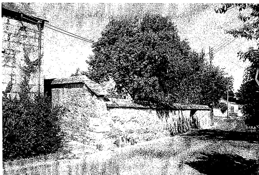
*Cob construction is found quite frequently in St. Tudy. Cob is usually built up on a stone plinth to protect it from rising damp, but also needs a good overhanging roof to protect it from wind and rain. Limewash or soft lime renders have traditionally been used to protect cob walls from erosion.*
