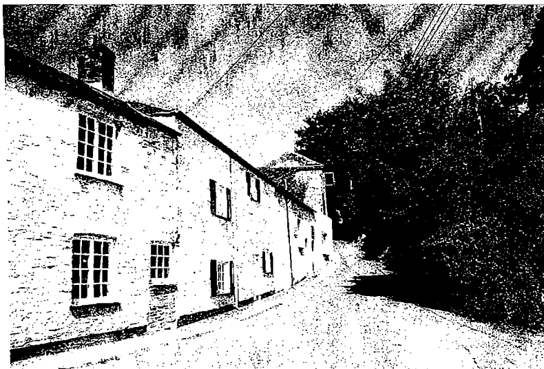
The road ascends steeply uphill from the bridge past the Social Club. Stone walls are often painted in white or cream in Lockett. Windows are usually small paned casements or sliding sashes.
