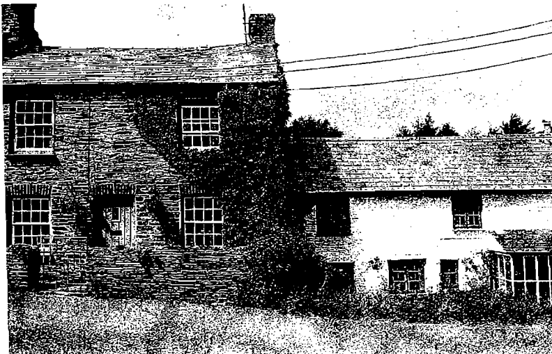
Close to Lockett Bridge, old, set down cottages indicate the original level of the road and ford, prior to the construction of the stone bridge. Later, taller, 19th century buildings are set higher, in response to the raised level of the carriageway.
