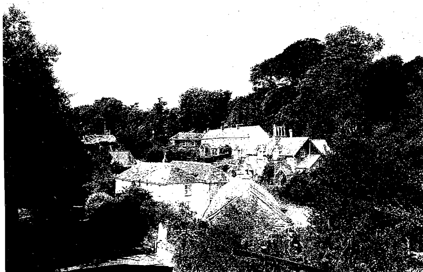
Mature trees form an important element of the bowl-shaped setting of the village.
