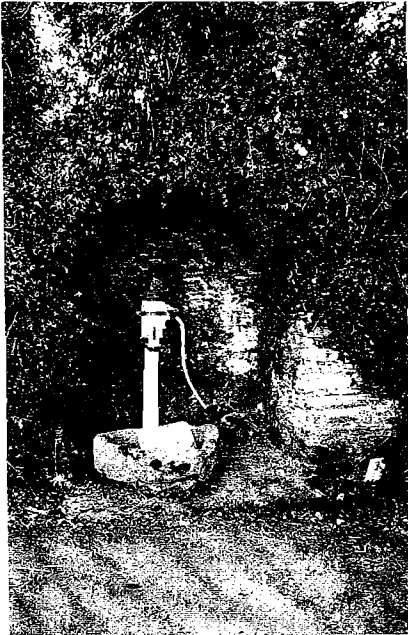
A 19th century iron pump and stone wellhouse is situated beside the lane leading uphill to Ballamminer's Farm.
